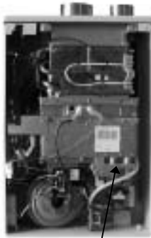
Manifold pressure tap
